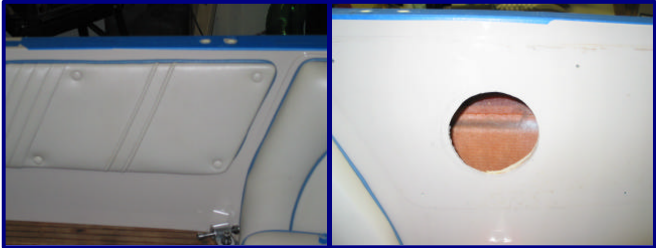
Figure 5 - Access to Underneath Deck
